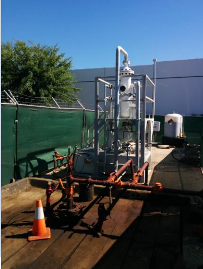
SandZapper 5K2D installed at the wellhead
